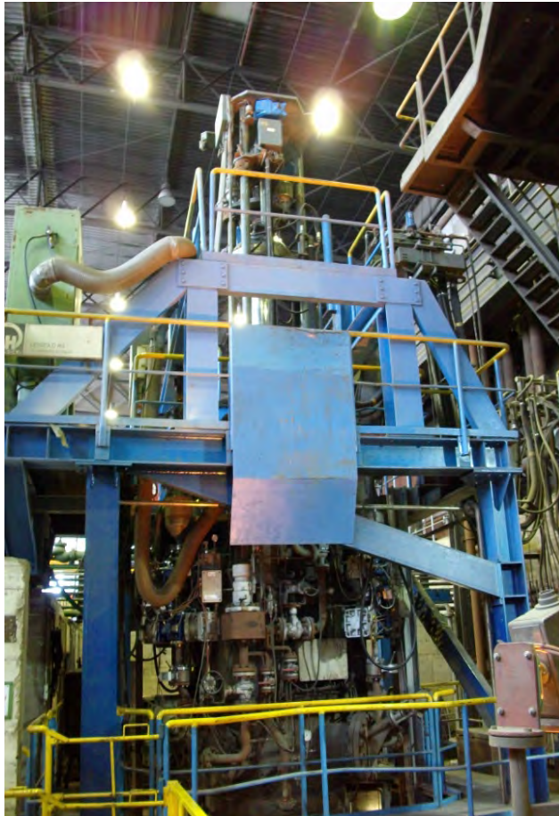
Fig. 3. View of the industrialized PESR -process at Energietechnik Essen GmbH for ingot weight up to 20 t und \varnothing 1030 mm.
